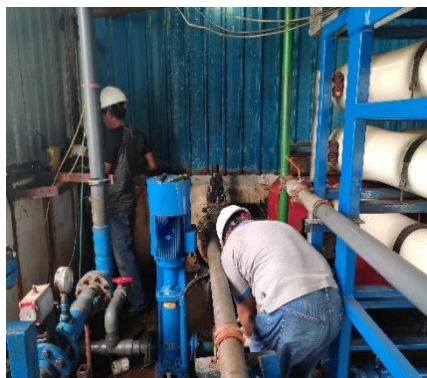
Gambar 6. Perawatan HP pump
